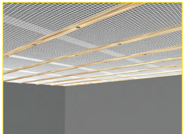
Fig.12: Fixed attachment of the sheets with the help of the slats - removing the auxiliary nails
