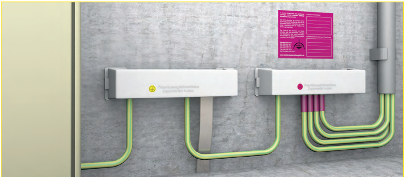
Fig. C2: Completed grounding of facade surfaces with labels
