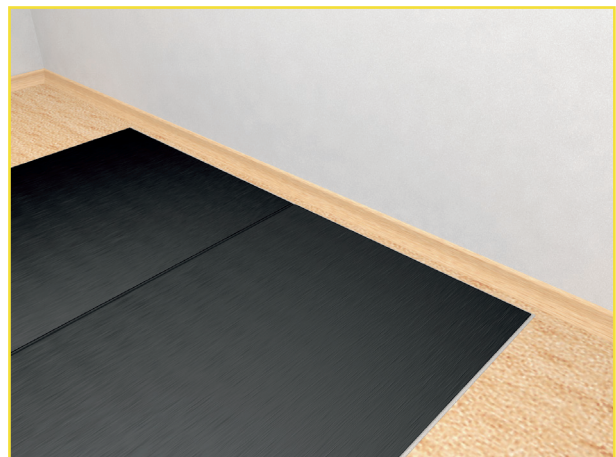
Fig.22: Laying out the screen material
