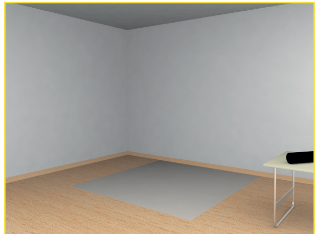
Fig.21: Laying out the underlay
