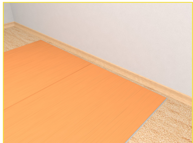
Fig.22: Laying out the screen material
